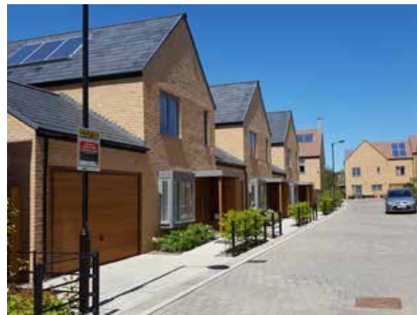
Photovoltaic panels, Trumpington Meadows, Cambridge
