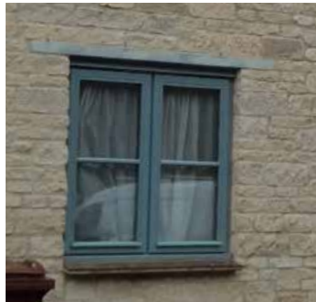
Casement window flush with wall, Bletchingdon
