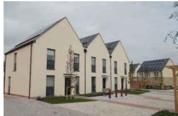
A shared surface street - NW Bicester
