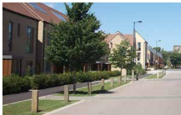
Incorporating SuDS along kerbside, Trumpington Meadows, Cambridge
