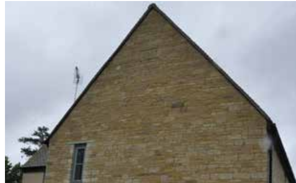
Steeply pitched roof with no overhang, Bletchington
